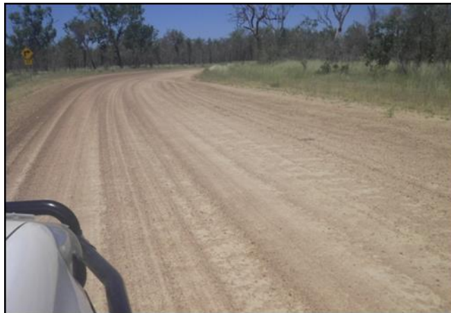
Figure - Gravel s-bend section north of Bora River Crossing
